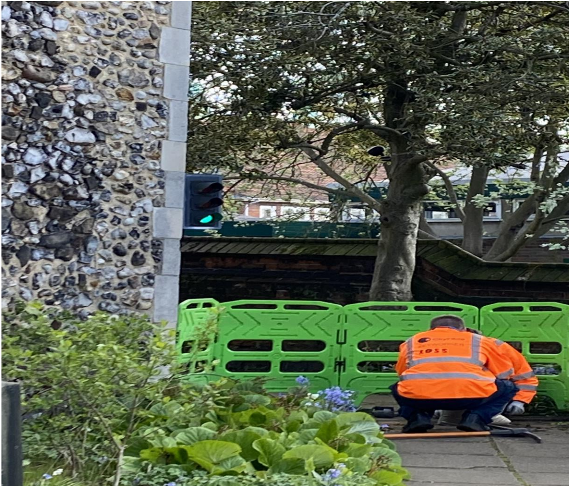
City Fibre installing broadband into the church this week.
